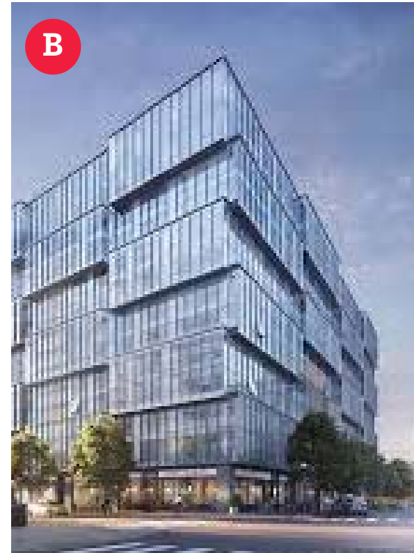
28 K St SE Glazing, Brick, Metal Panel
