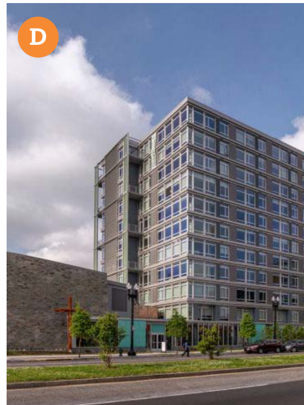
222 M St SW Glazing, Metal Panel
