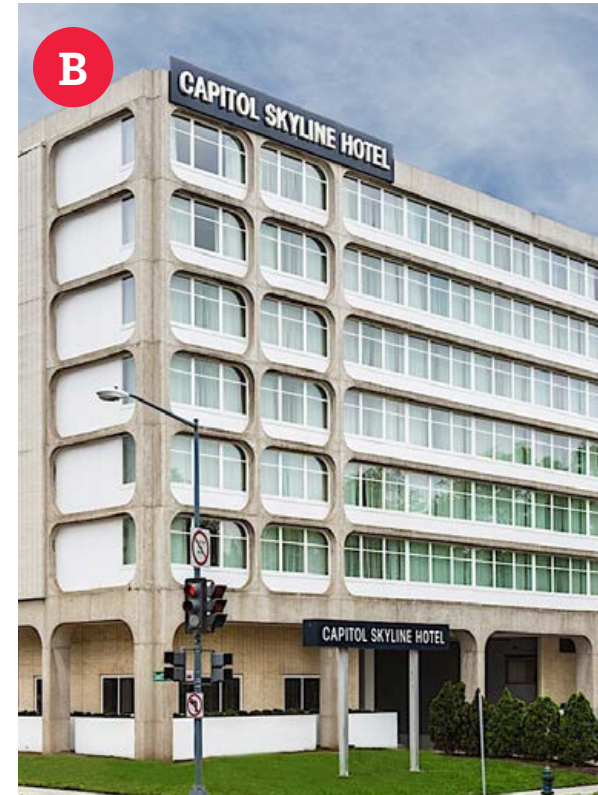
10 I St SW Concrete, Glazing
